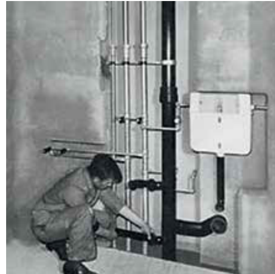
↑ Introducing the first concealed cistern in 1964
